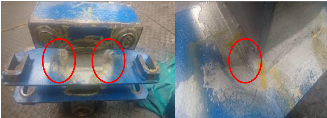
Reverchon Spinning Coaster cracking
