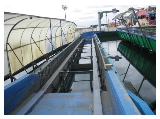
Initial investigations suggest that the passenger unit (log) involved was released following a temporary halt for technical reasons, and then failed to slow down to a safe residual speed in the water tank. This resulted in the passengers being ejected from the log.
