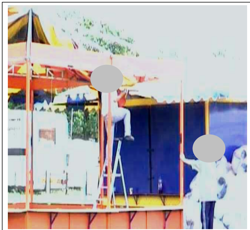
FIGURE 21 INADEQUATE WORKING PLATFORM
