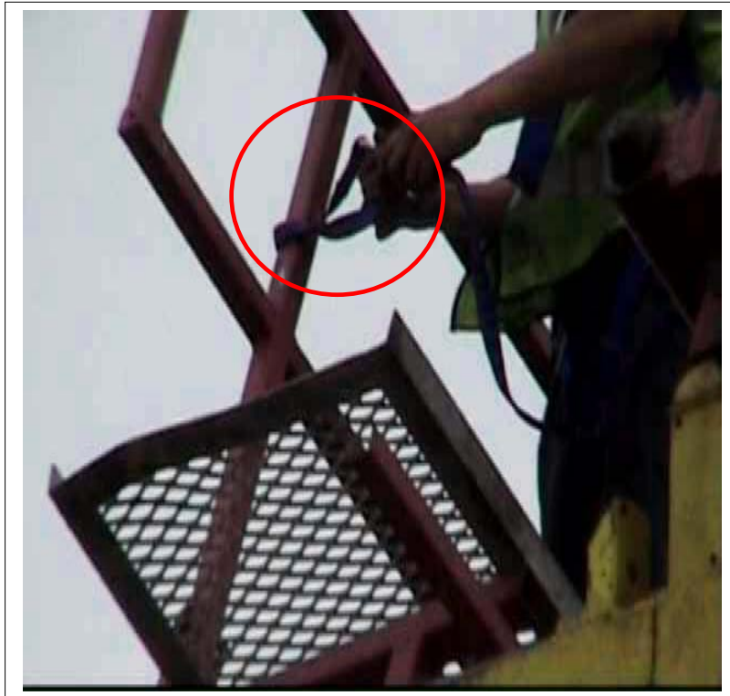
FIGURE 31 ANCHORING OF PPE ON GUARDRAILS
