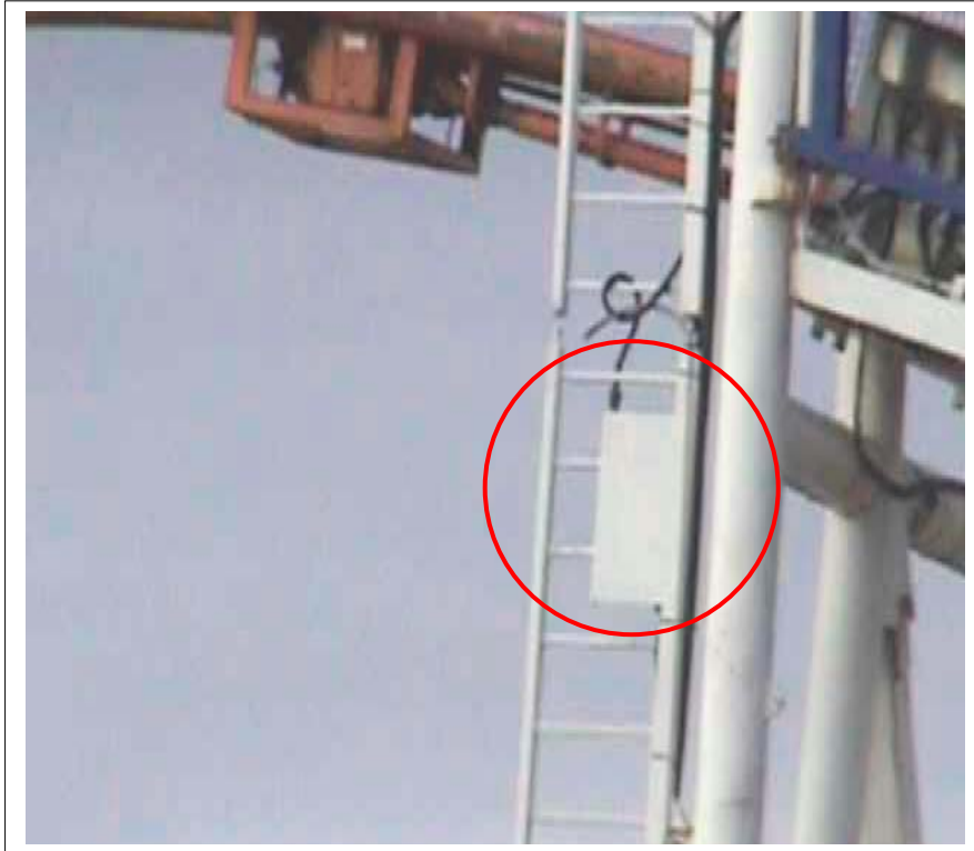
FIGURE 3 FIXED LADDER INTERRUPTIONS/OBSTRUCTIONS
