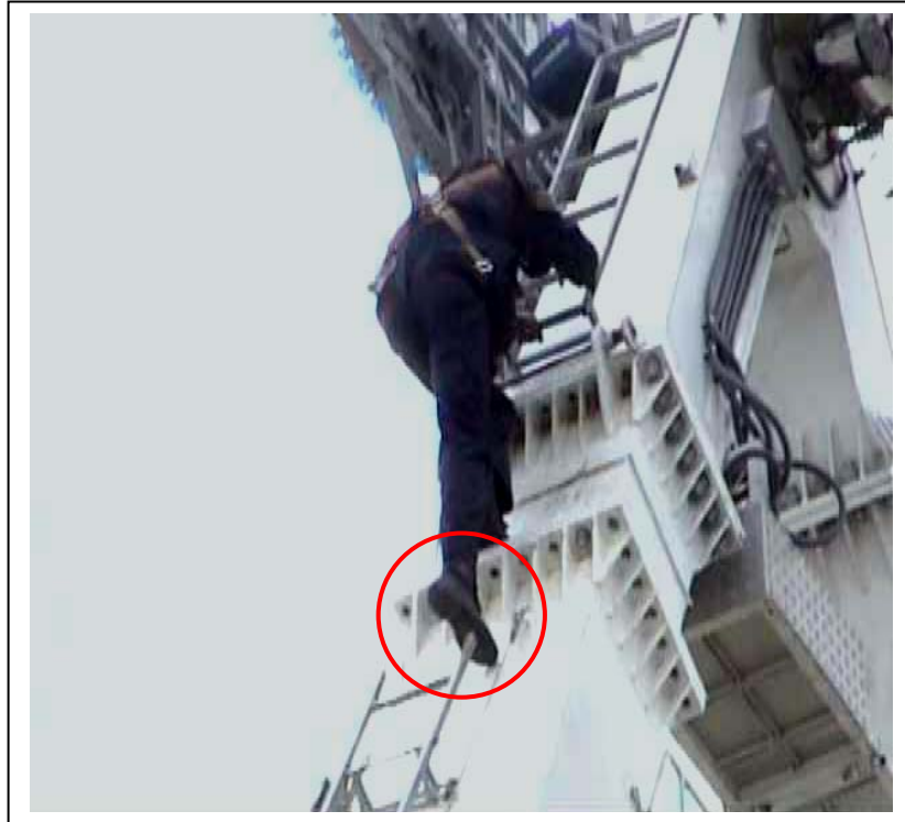
FIGURE 1 INADEQUATE FOOT-HOLDS AND HAND-HOLDS AT OVER 100 METRES
