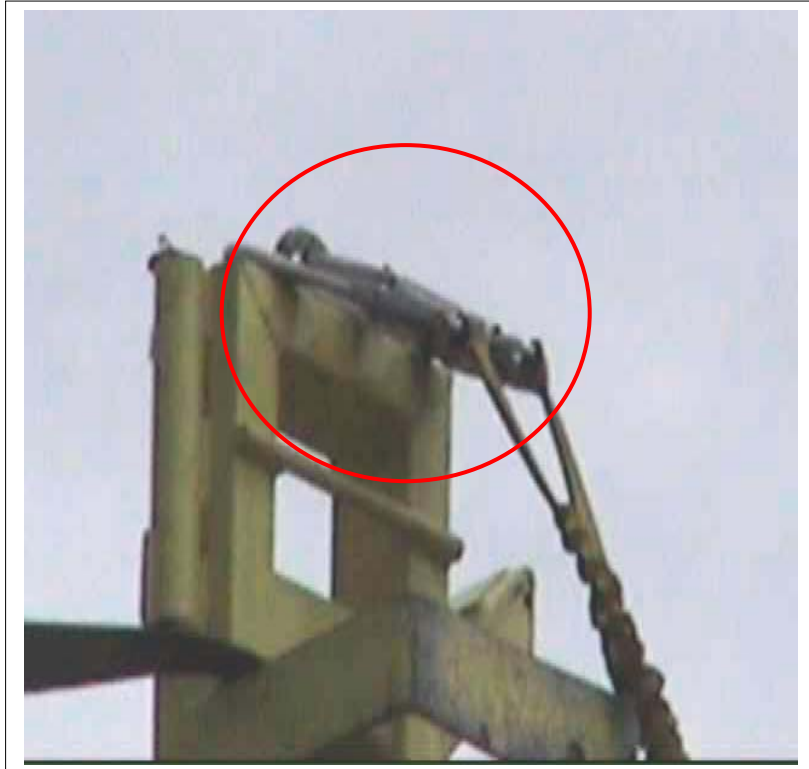
FIGURE 37 POOR ANCHORING TECHNIQUES
