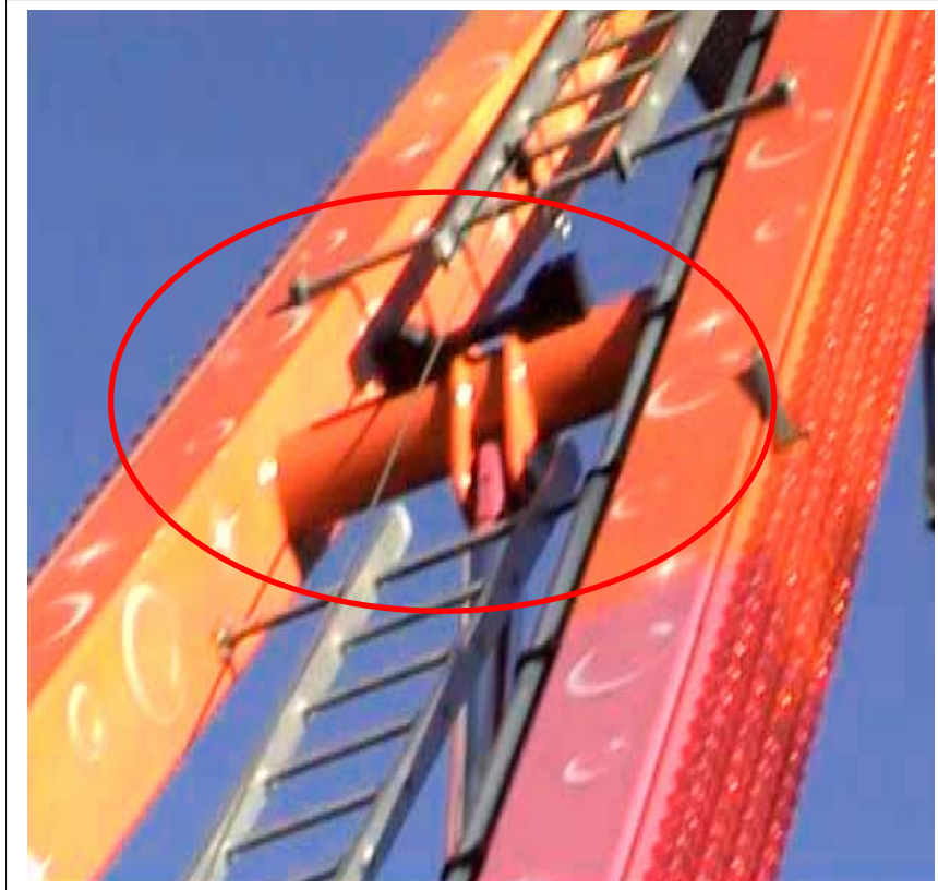
FIGURE 5 FIXED LADDER INTERRUPTIONS/OBSTRUCTIONS
