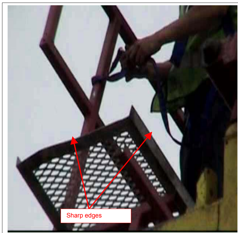
FIGURE 26 POTENTIAL FALL HAZARD - SHARP EDGES
