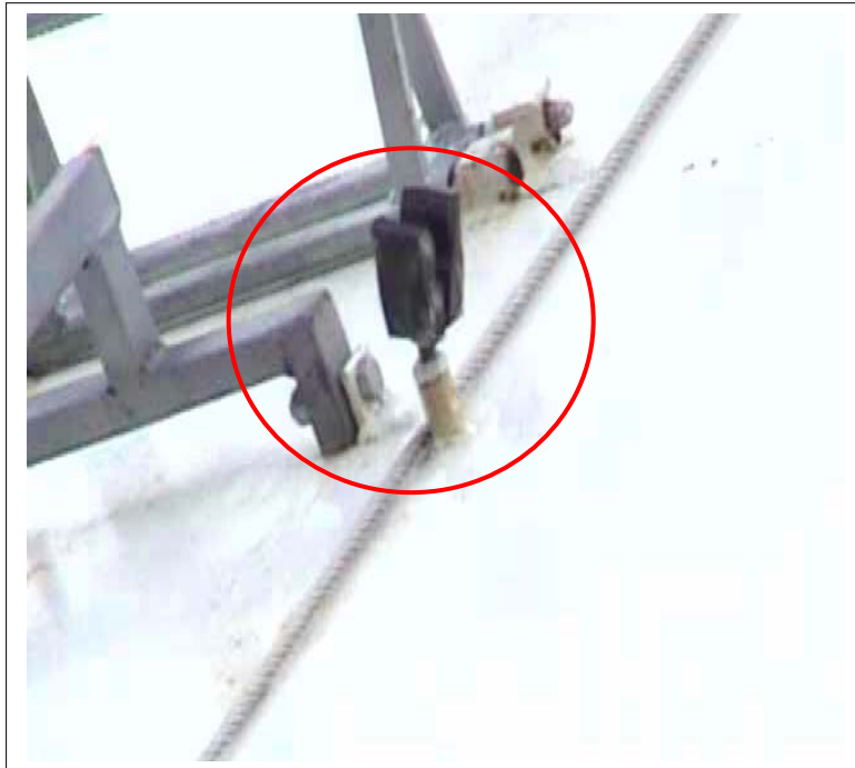
FIGURE 33 DEFORMED UNUSED FALL ARREST CABLE GUIDE
