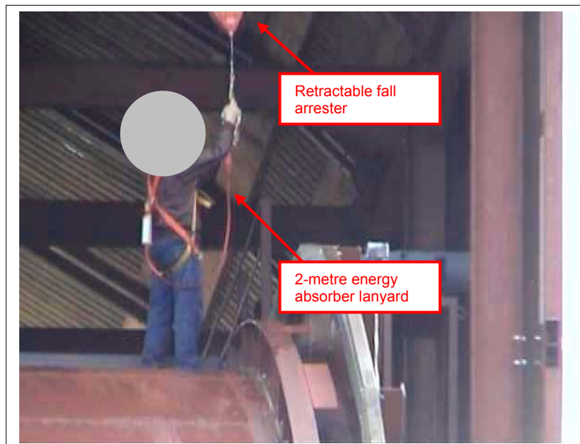
FIGURE 42 ENERGY ABSORBER LANYARD CONNECTED IN SERIES WITH A RETRACTABLE TYPE FALL ARRESTER
