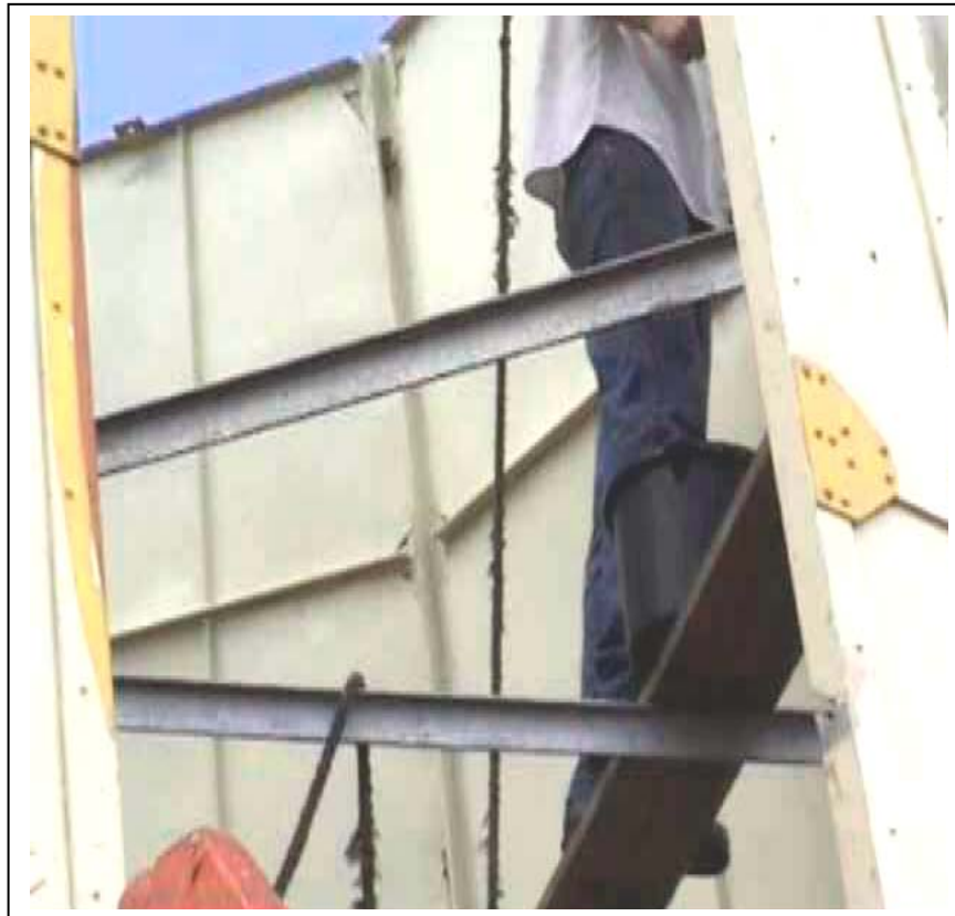
FIGURE 15 INADEQUATE UNSECURED WORKING PLATFORM
