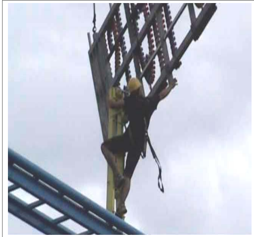
FIGURE 22 MAN-HANDLING OF EQUIPMENT INTO POSITION
