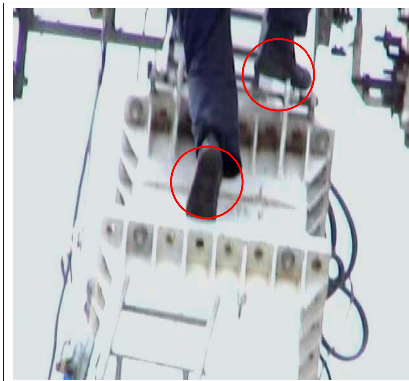
FIGURE 2 INADEQUATE FOOT-HOLDS AND HAND-HOLDS AT OVER 100 METRES
