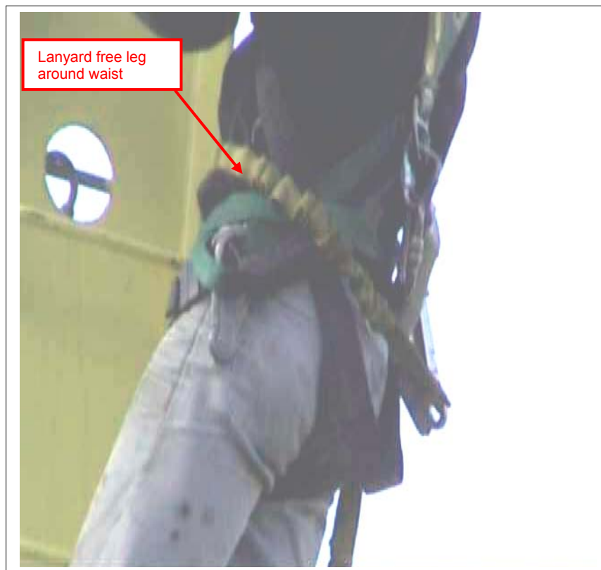
FIGURE 41 FREE LEG OF TWIN ENERGY ABSORBER LANYARD TIED AROUND WORKERS WAIST
