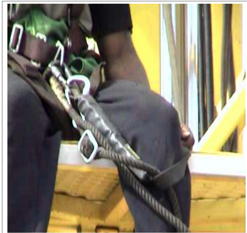
FIGURE 40 POOR ADJUSTMENT OF HARNESS WITH ATTACHMENT POINT POSITIONED AT THE WAIST
