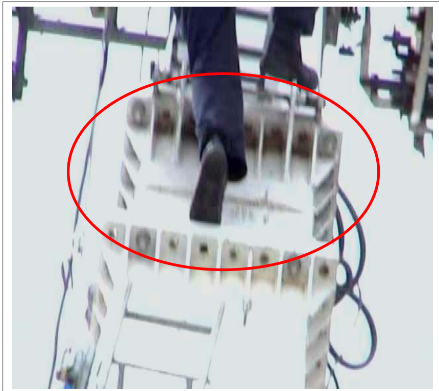
FIGURE 6 FIXED LADDER INTERRUPTIONS/OBSTRUCTIONS
