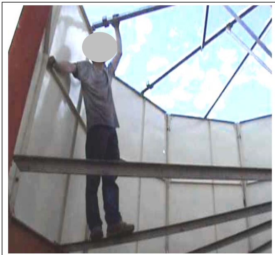
FIGURE 16 INADEQUATE WORKING PLATFORM
