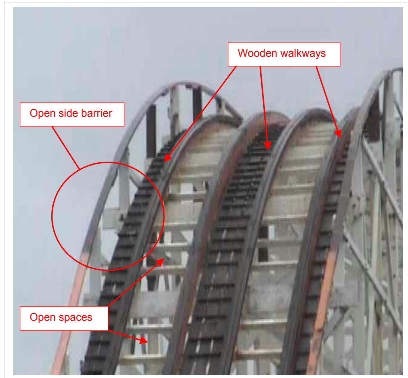
FIGURE 9 INADEQUATE WALKWAYS
