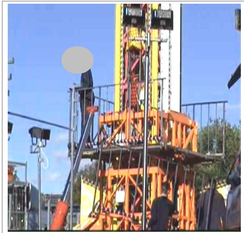
FIGURE 14 INTEGRATED WORKING PLATFORM WITH FALL PROTECTION
