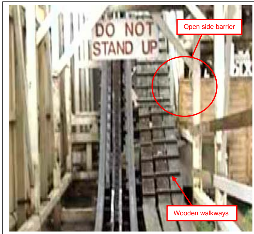
FIGURE 7 INADEQUATE WALKWAYS
