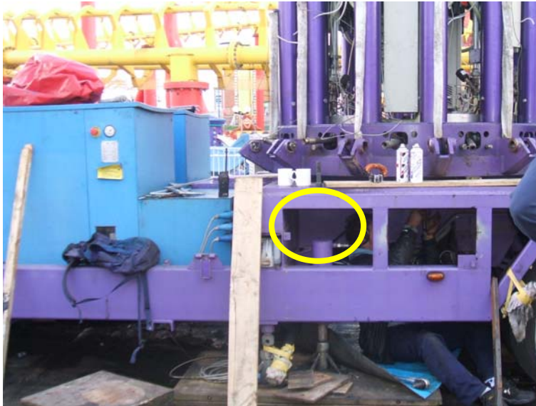
2. 1Location of cracking under the slewing ring.
